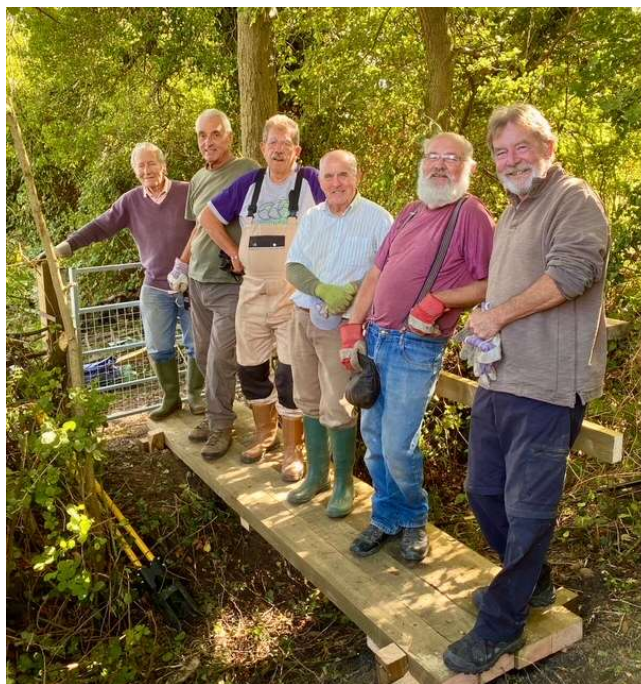
New Gate & Ditch Crossing Installation – 'The Slinget'
