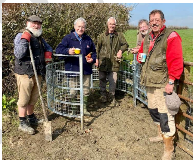
Latest Kissing Gate installation beyond Back Lane
